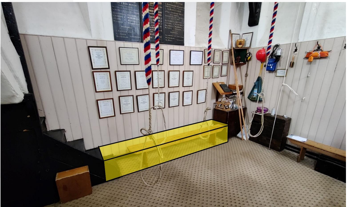
Mock-up showing proposed winch boxing in bell ringing chamber (exact dimensions subject to further investigation)
